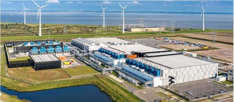
[Google Data Center, Eemshaven, Netherlands]
